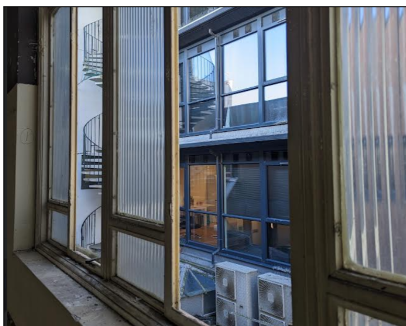
Figure IV - view of the rear of Worthing House
